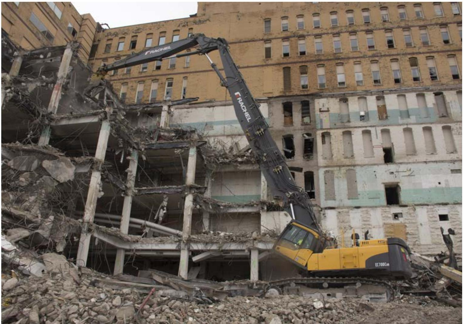
**Volvo EC700C HR High Reach Demolition Excavator**
