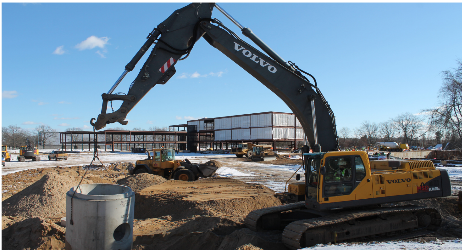
The workhorse of Glenn's fleet is his 2002 EC460B crawler excavator, seen here placing a concrete manhole section at the New Windsor magnet school project.
