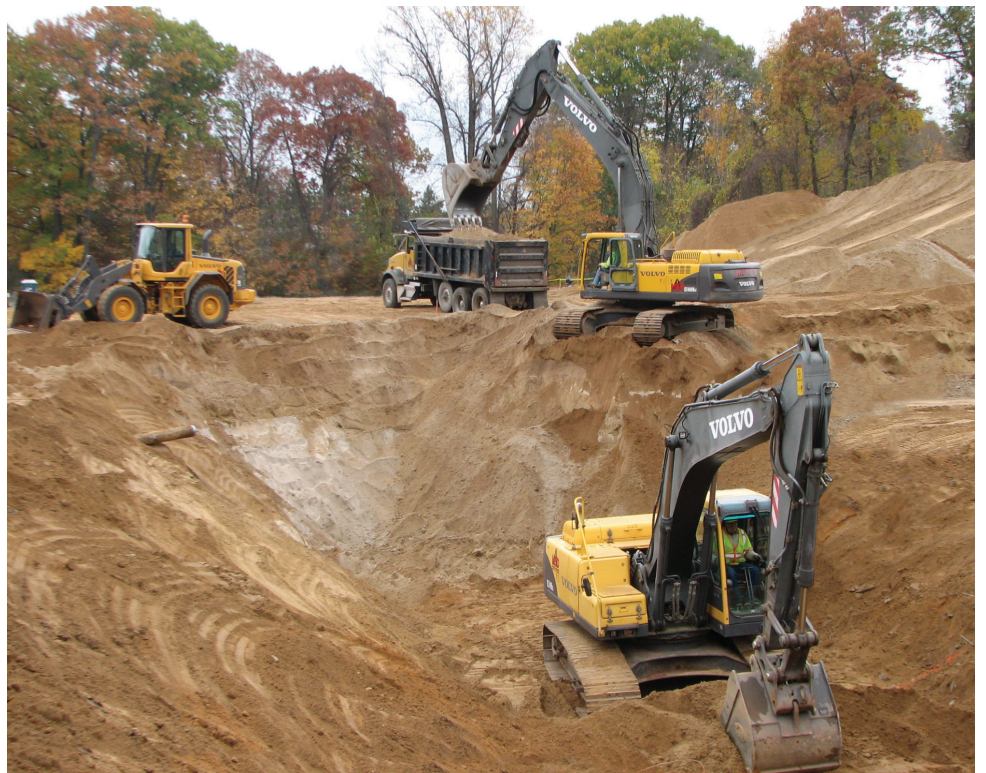
For the New Windsor magnet school project, MSD was contracted to build a 30' deep retaining wall, foundation excavation, install water/sewer/storm drainage, and slab and pavement prep.
