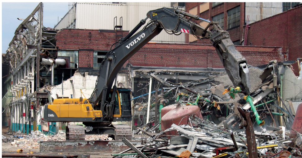
Scrap is sorted during demolition and processed on site.
