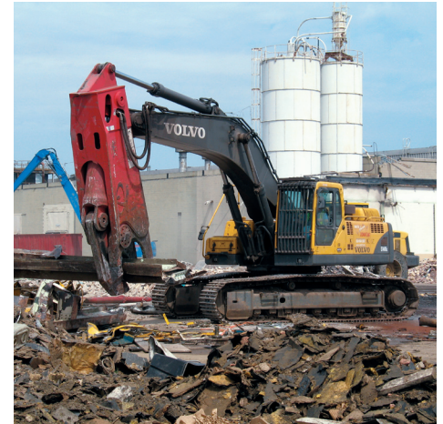
This specialized shear attaches directly to the boom for strength.
