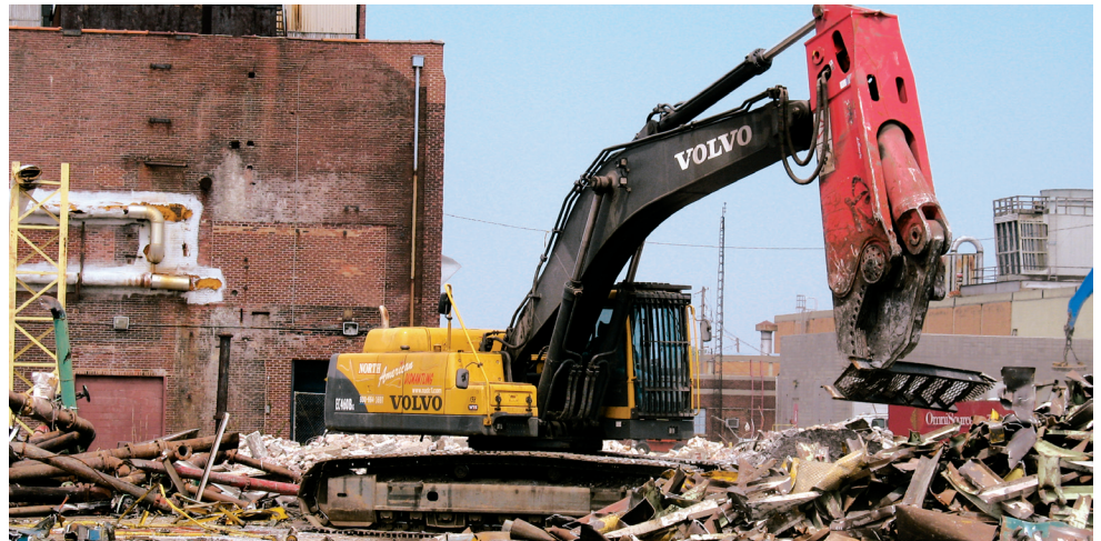
Piece by piece, Volvo and a shear attachment cut this factory down to size.
