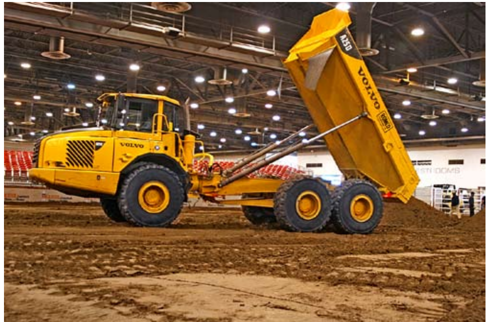
A Volvo articulated hauler moves dirt into the arena at Reliant Park for the 2010 Houston Livestock Show and Rodeo.
