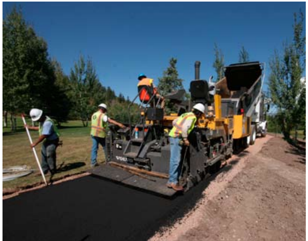
Adding asphalt paving services in addition to excavation gives Trulove a competitive edge.
