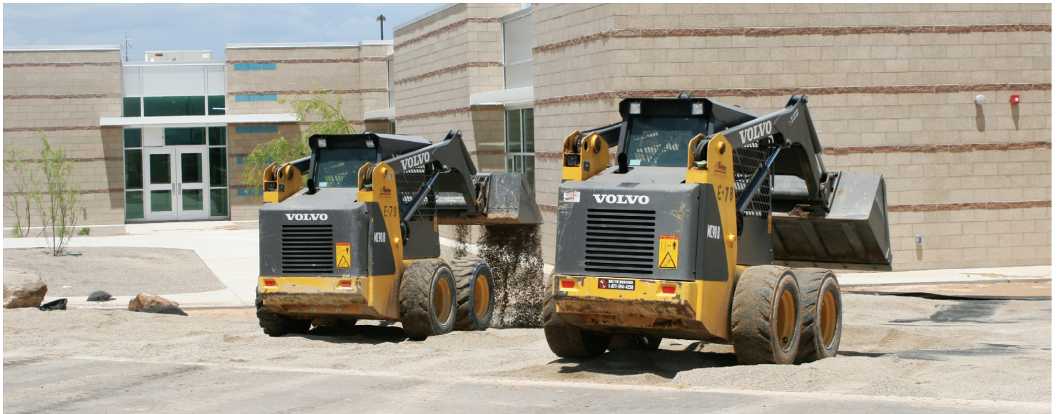
Two of Accent's Volvo skid steer loaders load and carry crushed fines for landscaping at an elementary school in Rio Rancho, New Mexico.
