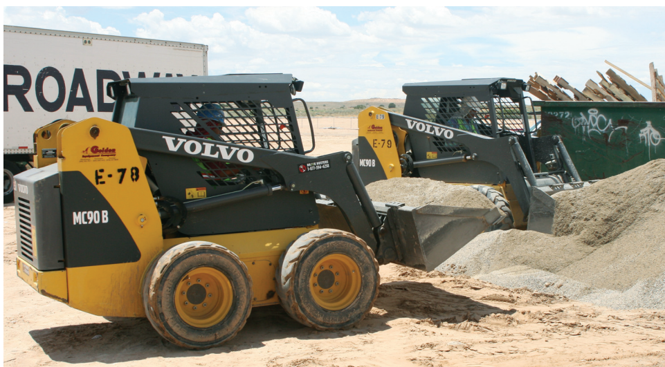
Two skid steer loaders load crushed fines for use in landscaping an elementary school in Rio Rancho, N.M.
