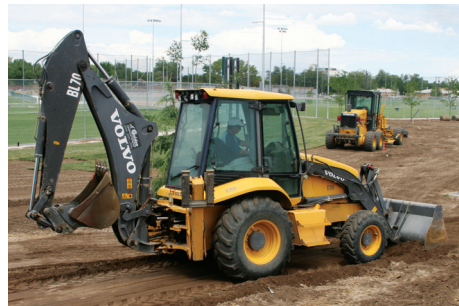
A Volvo BL70 backhoe puts the finishing touches on the grade at Tingley Park in Albuquerque, N.M.
