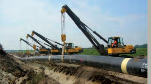
Pipelaying is a real team effort. Thanks to the boom mounted light bars – an integral part of the unique, Load Management System – the lowering-in foreman and other operators on the line can effectively monitor the management of the load and react accordingly.
