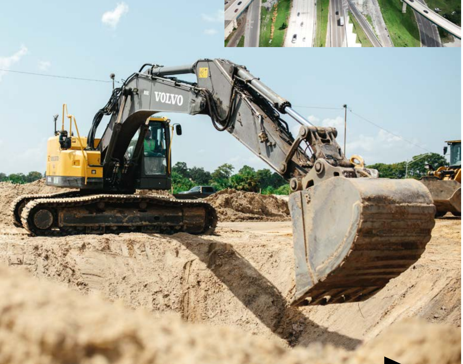
01 Motorists make more than 1.5 million trips on Florida's Interstate 4 every day. 02 Typical tasks for the Volvo excavators include digging trenches and loading trucks.
