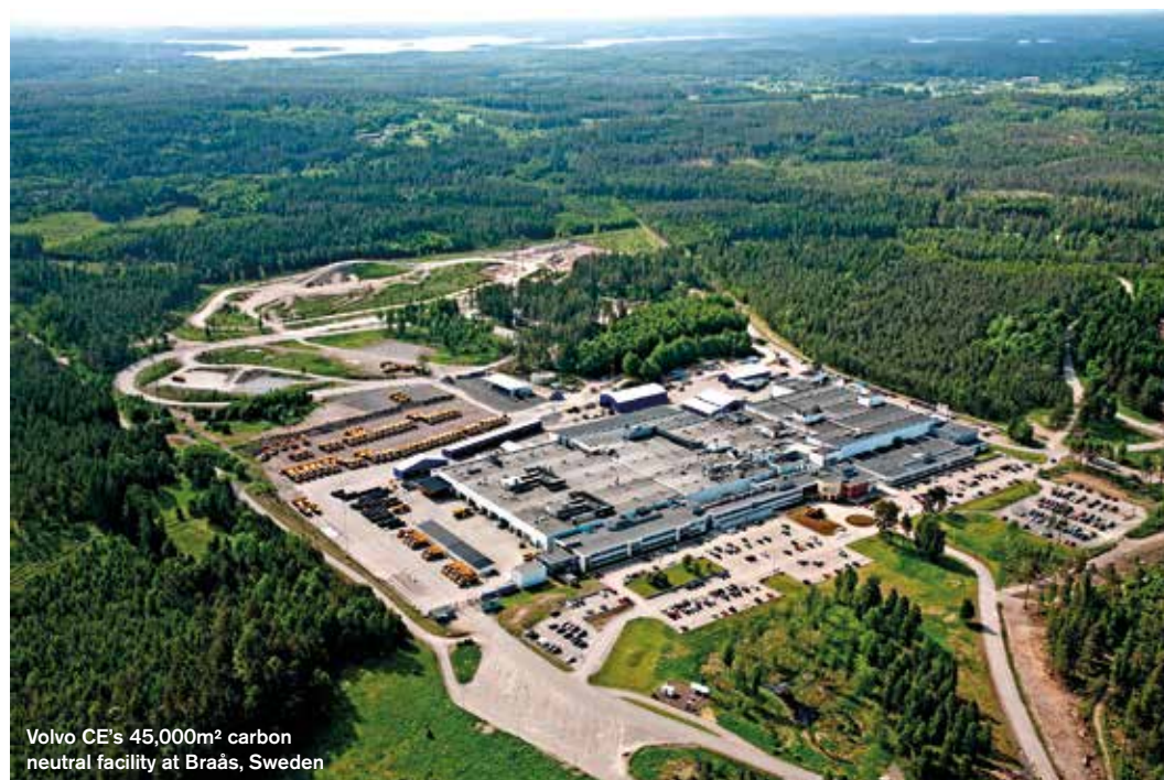
The articulated hauler facility at Braås in southern Sweden relies entirely on renewable energy sources
