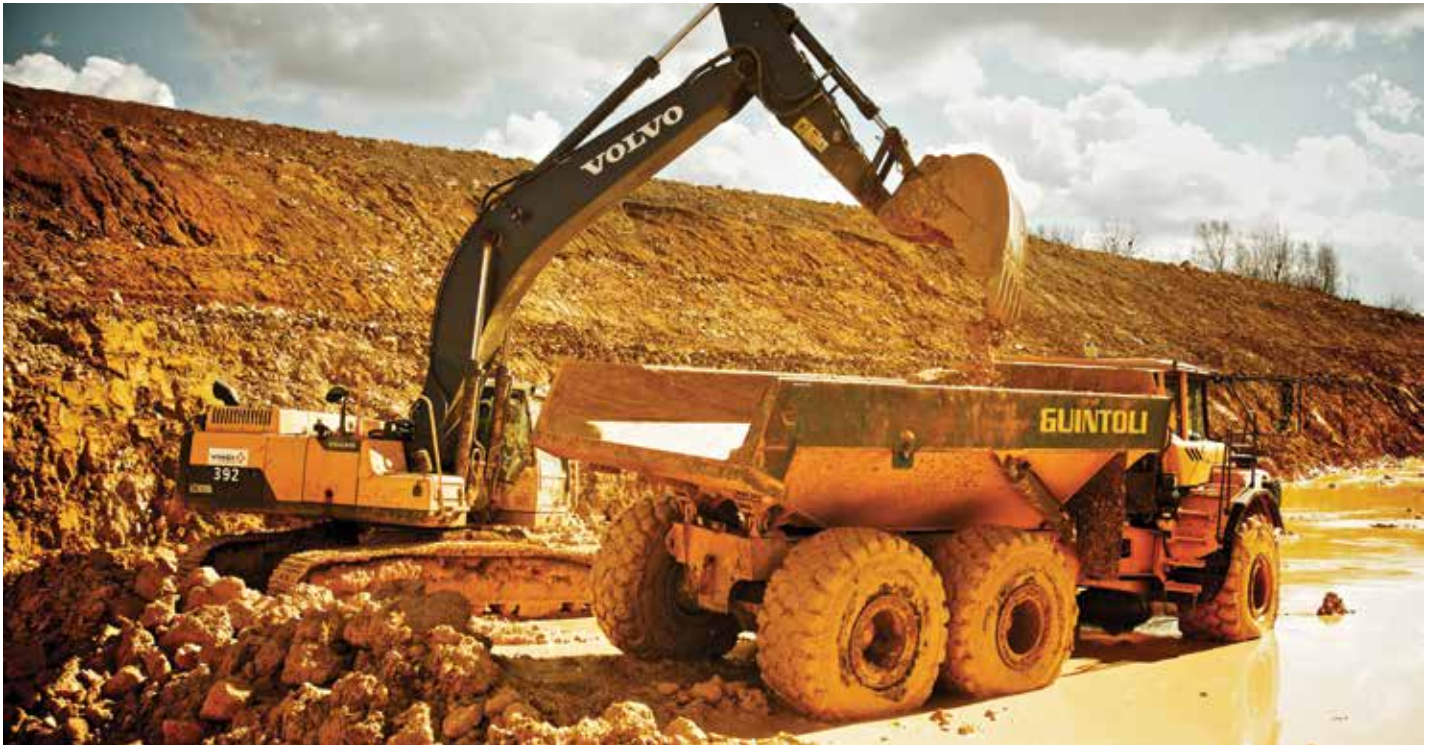
The Volvo machines are working in some very challenging conditions and coping very well.
