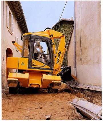
"9.25 am. Backfilling of the trench. Clunk Click, the bucket was in place and I switched to "loader" mode. With my left hand on the steering wheel and my right hand on the manipulator where all the controls are grouped together, I appreciated the flexibility of the machine which makes it possible to work with an offset and to pivot 360° despite the narrowness of the street."
