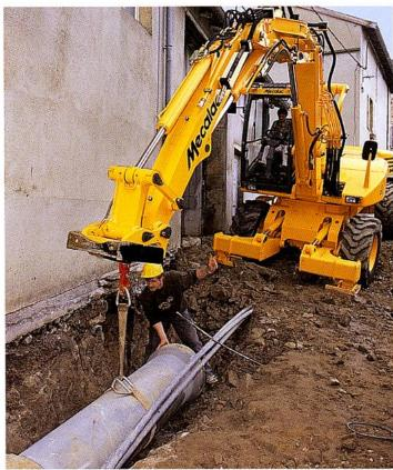
"8.50 am. Gentle positioning and fitting of a pipe.
