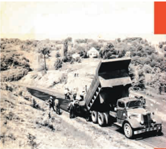
Handling 15 ton trucks on a 12% grade on Pennsylvania County work.
