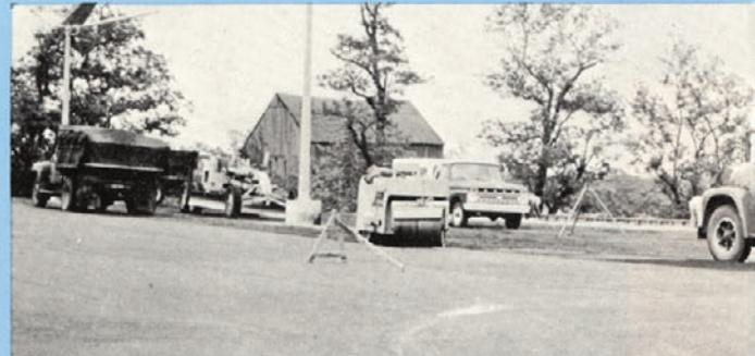
The PF-25 is ideal for paving streets, driveways and similar projects where maneuverability and versatility are important. By simply removing screed extensions, the PF-25 is under the 8-foot legal width—It is not necessary to remove screed side arms or other parts. A 24 mph travel speed gets
