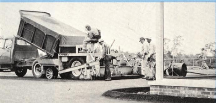
it from location to location with a minimum of down time; in many cases as fast as trucks. Its small size lets it work in tight places with ease; paving widths from six to eleven feet and paving speeds from 15 to 60 fpm give extra flexibility and versatility not available with crawler machines.
