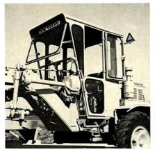
The reverse rake of the windscreen gives the driver a good view of the operating gear and the roof overhang serves as sun-visor. The windscreen and top section of the doors can be locked in the open position.
