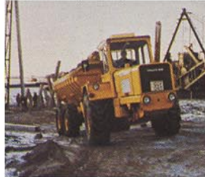
Bridge construction, Sweden
