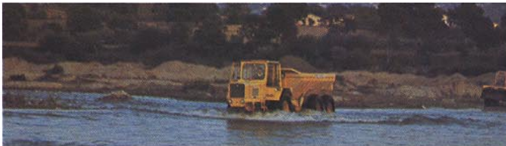
Transport of river bed gravel, Italy
