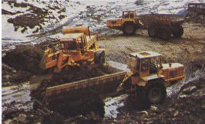
Construction of power station dam, Austria
