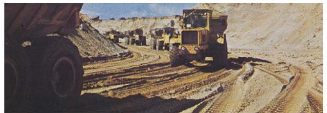
Road construction, Holland
