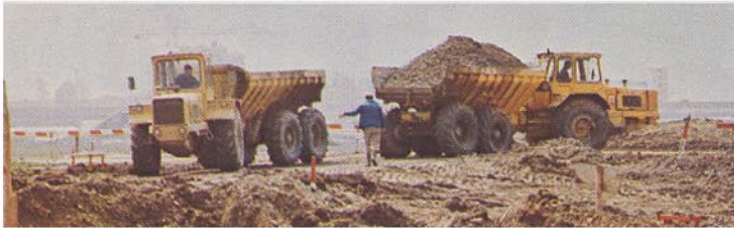
Airport construction, Switzerland
