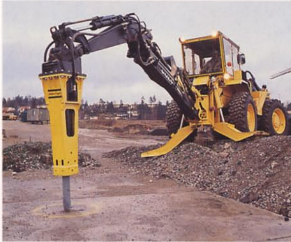
Maintenance and repair of gravel roads.
