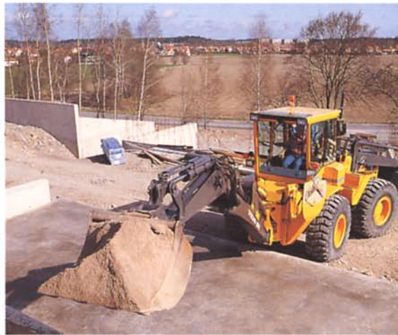
Handling materials on a building site.
