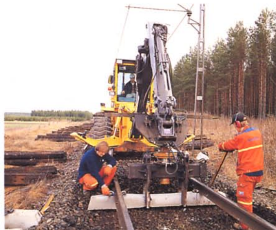
Replacing railway cross-ties.
