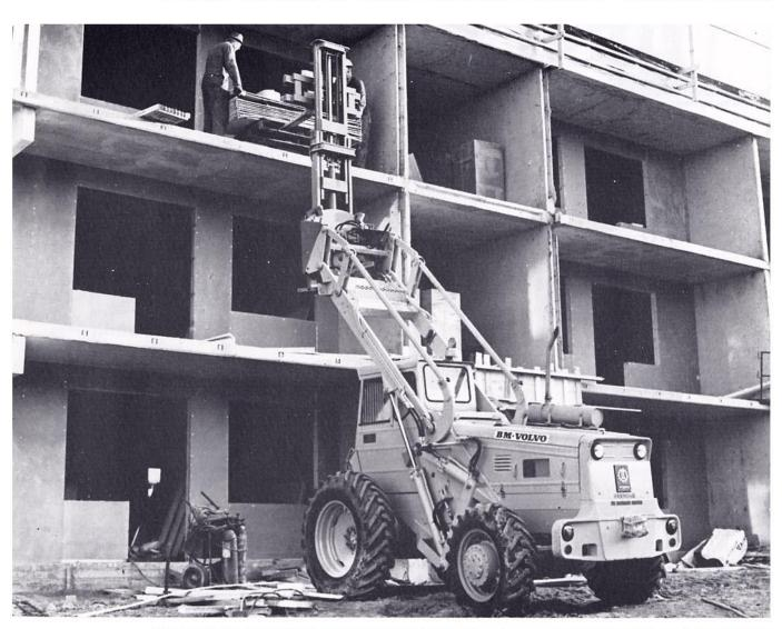
The VOLVO BM Hi-Lift — a new forklift attachment which gives greater flexibility and cuts the cost of materials handling. A VOLVO BM "Allrounder" loader, fitted with the Hi-Lift forms a mobile and highly flexible unit for off-the-road transport. It gives a precision lift up to a height of 23 ft (7 m). The Hi-Lift therefore supplements and, in many cases, replaces conventional equipment and methods in the handling of palletized
