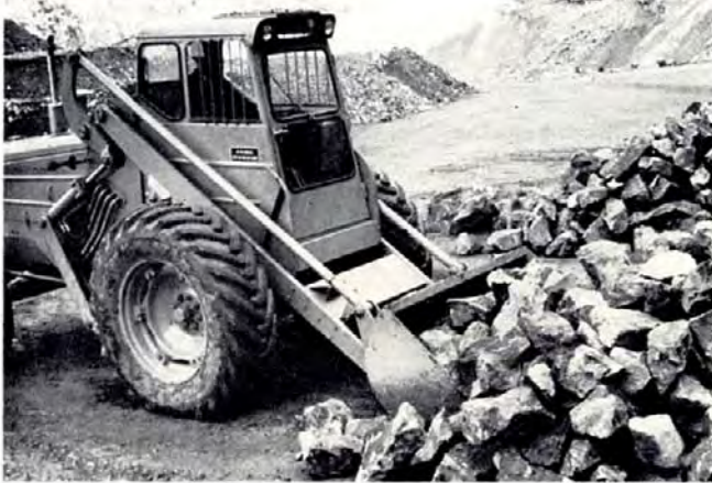
Mucking natural and blast quarry rubble, with sheet or open mucking scoop.
