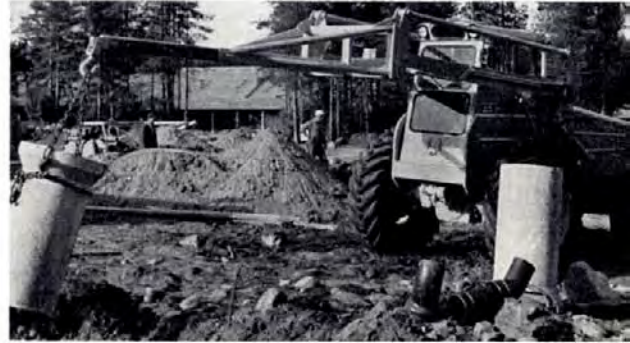
Pipelaying, materials handling and machine removals on construction sites, using the extendable crane jib.
