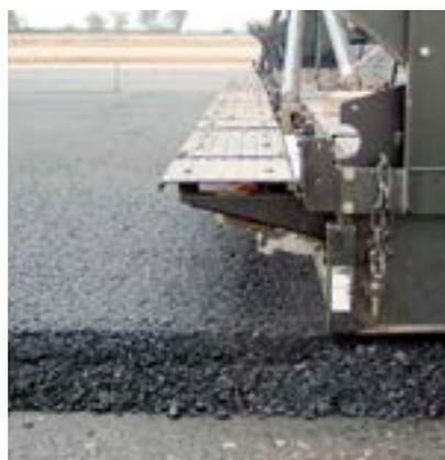
Volvo Duotamp high-compaction screeds have proved their worth in applications all over the world, e.g. paving base, binder and wearing courses, granular materials, CBM, RCC, and even in special applications such as the laying of bituminous sealing surfaces on dam slopes and high banking vehicle racing and testing circuits, where traditional methods of compaction cannot be used.
