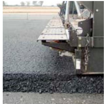
Volvo Duotamp high-compaction screeds have proved their worth in applications all over the world, e.g. paving base, binder and wearing courses, granular materials, CBM, RCC, and even in special applications such as the laying of bituminous sealing surfaces on dam slopes and high banking vehicle racing and testing circuits, where traditional methods of compaction cannot be used.
