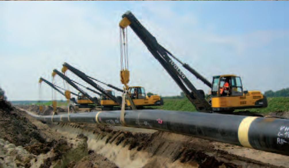
Pipelaying is a real team effort. Thanks to the boom mounted light bars – an integral part of the unique, Load Management System – the lowering-in foreman and other operators on the line can effectively monitor the management of the load and react accordingly.
