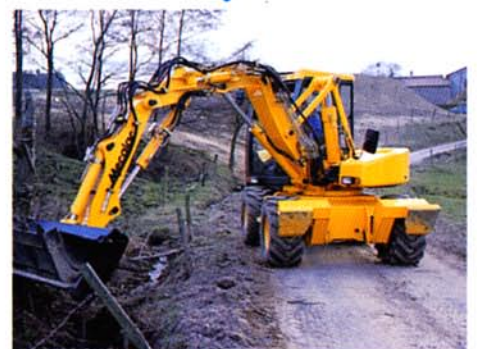
Working over an obstacle using a 4-in-1 bucket.
