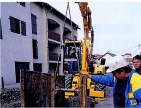
Handling heavy liners, face on...
