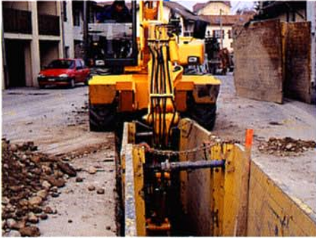
Flexibility and depth in excavation
