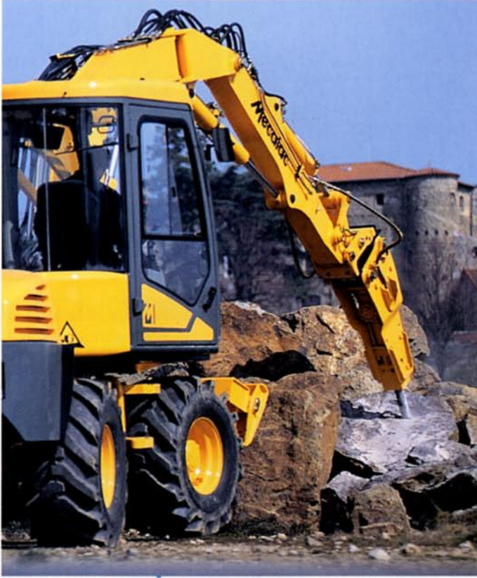
Hydraulic rock-breaking work
