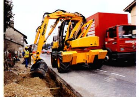
Rehandling material above a trench
