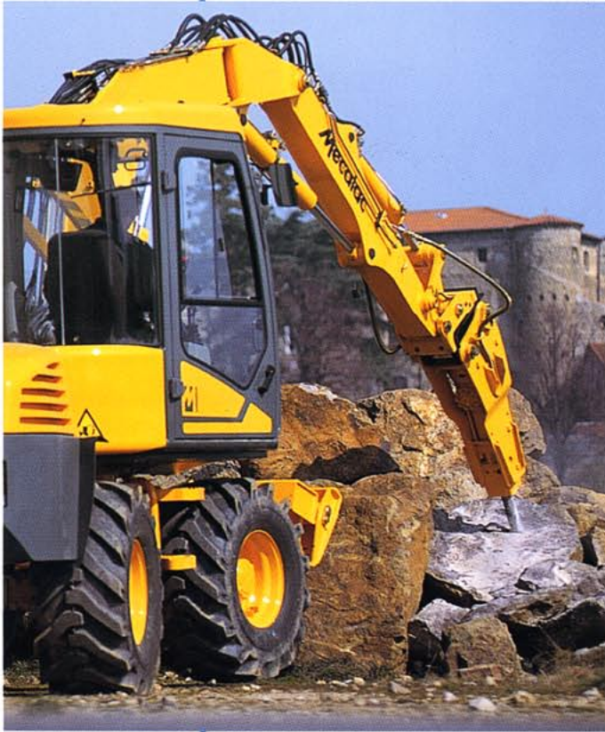
Hydraulic rock-breaking work
