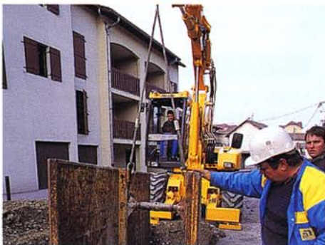
Handling heavy liners, face on...
