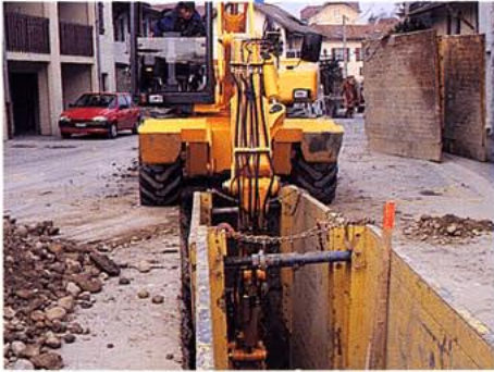
Flexibility and depth in excavation
