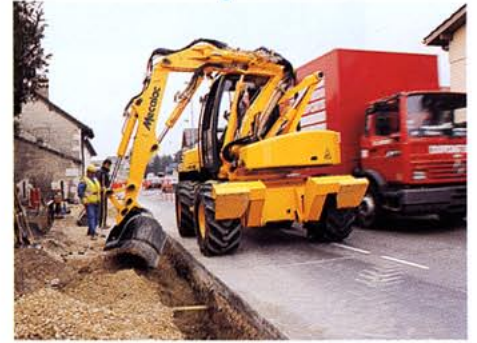
Rehandling material above a trench
