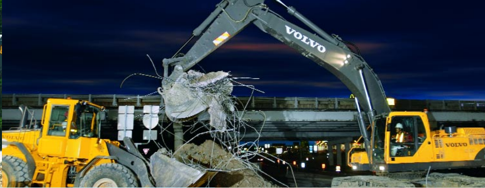
Control: Hydraulics allow precision placement
