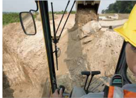
Attachments: Buckets, hammers, compaction
